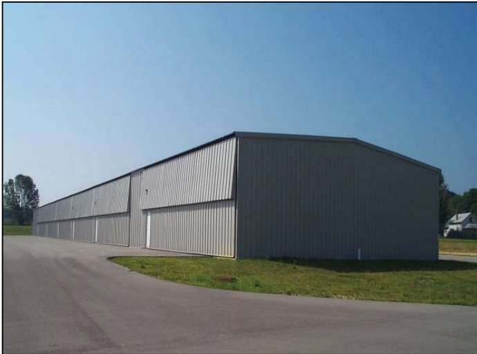
SOURCE: Monroe County Airport.
