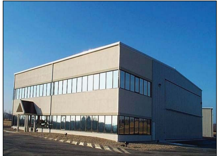
SOURCE: Monroe County Airport.
