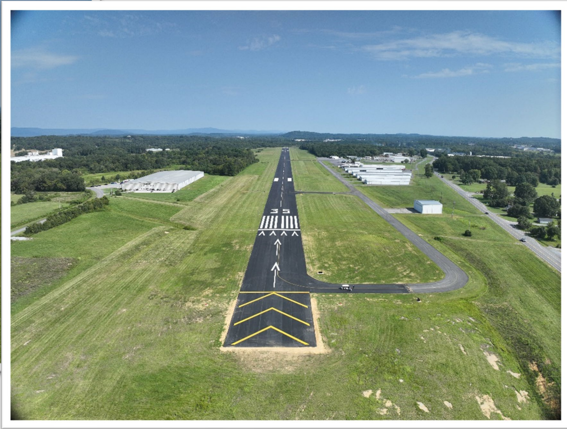
Tom B David Field Rehabilitate Runway 17/35 Total Construction Cost: $2,686,003
