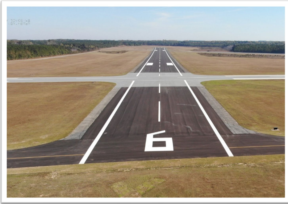
Statesboro-Bulloch County Airport Rehabilitate Runway 6-24 (Crosswind Runway) Total Project Cost: $1,616,479
