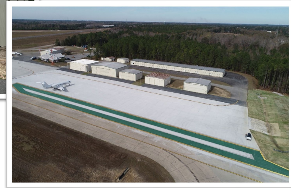
Vidalia Regional Airport Apron Expansion Total Project Cost: $3,645,513
